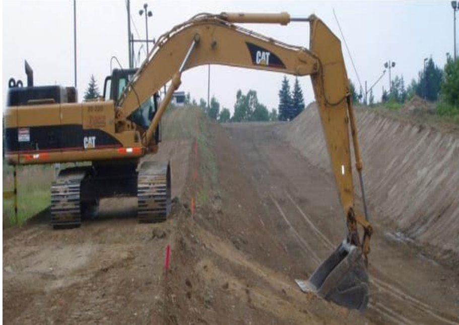
Figure 10 Compacted Earth Lining
