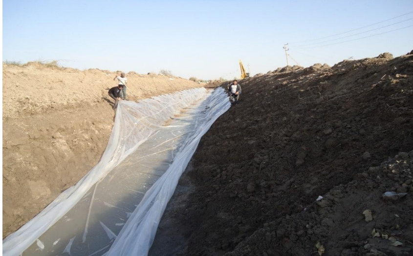
Figure 15 Plastic lining
