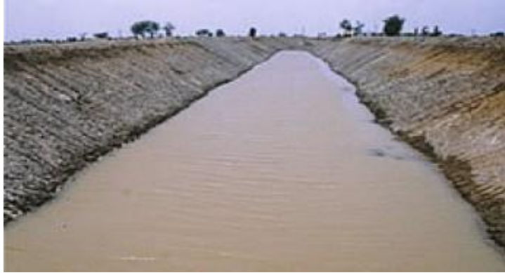
Figure 14 Boulder lining
