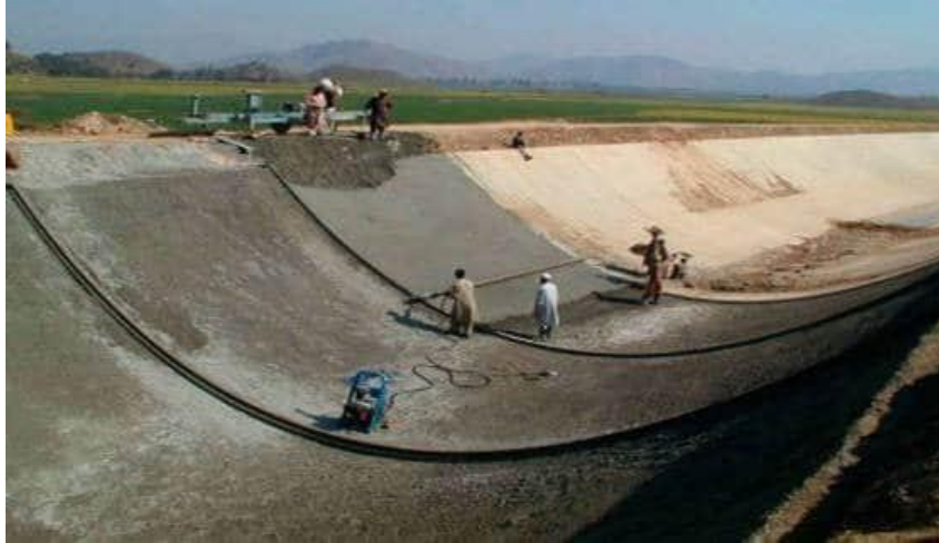
Figure 12 Cement Concrete lining
