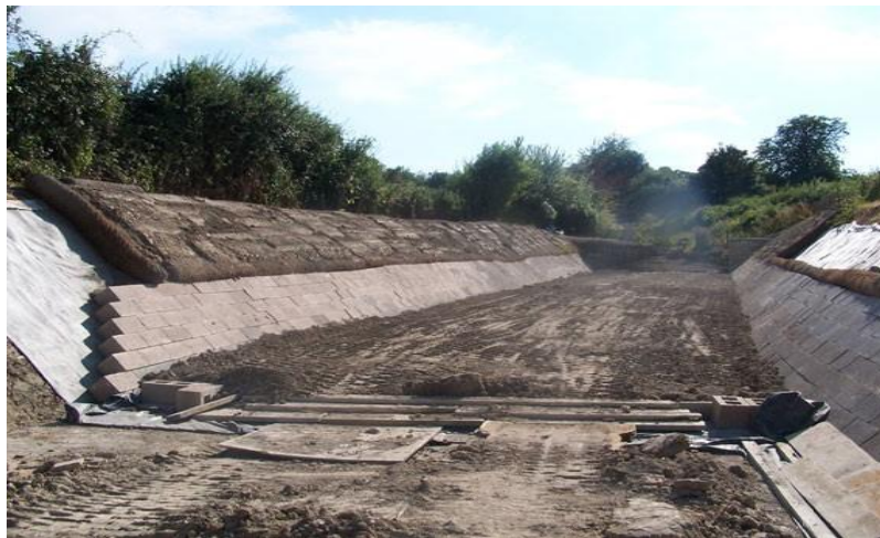
Figure 13 Brick lining
