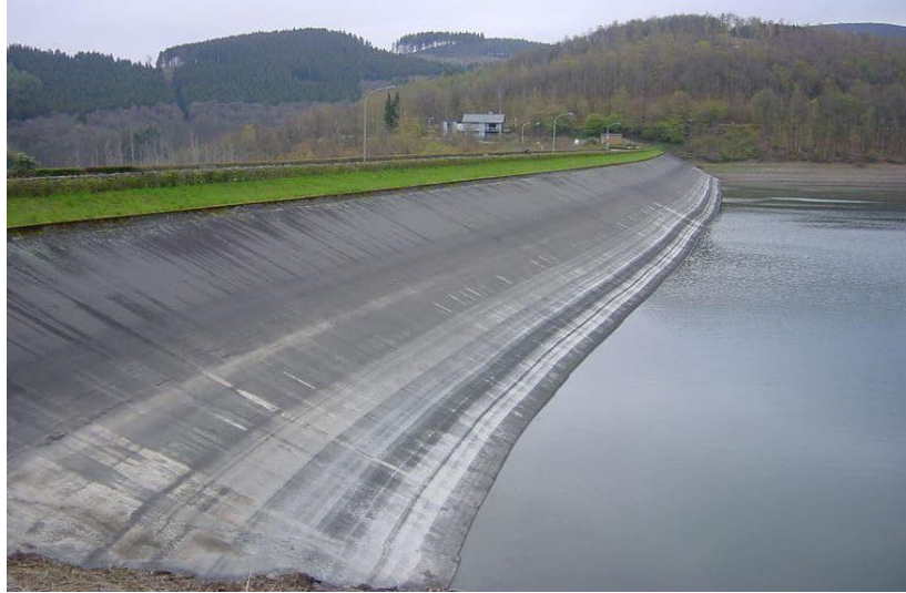
Figure 11 Soil Cement lining
